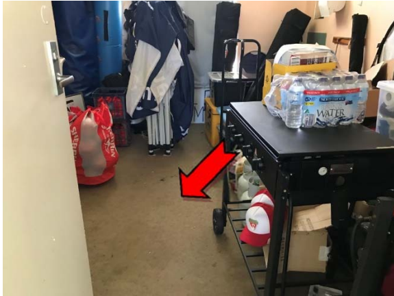
Photo 13. Interior, room 2, beneath carpet, throughout – assumed asbestos-containing vinyl floor tiles.
