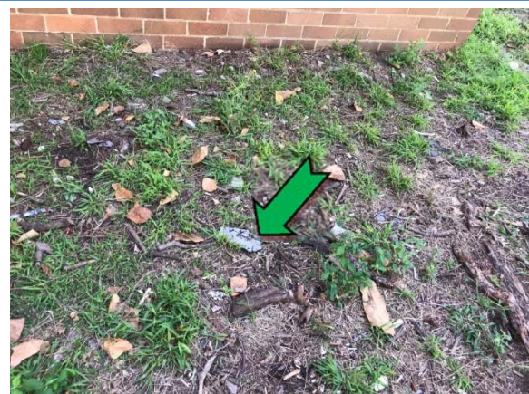
Photo 6. Exterior, west elevation, ground, debris – non asbestos-containing bituminous material.
