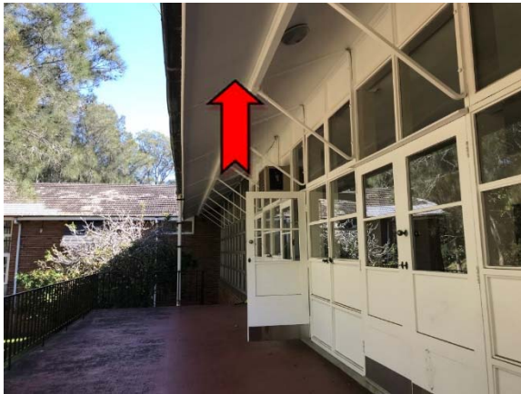
Photo 3. Exterior, western elevation, awning – assumed asbestos-containing fibre cement sheeting.
