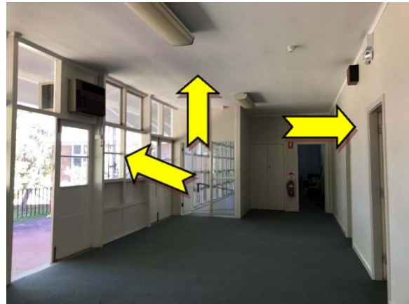
Photo 22. Interior, throughout, walls, window frames and ceiling – suspected lead-containing white upper paint systems.
