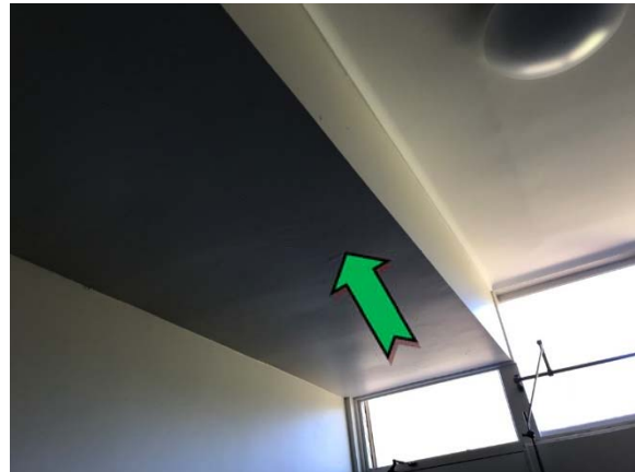
Photo 10. Interior, male toilets, high level boxing – non asbestos-containing fibre cement sheeting.
