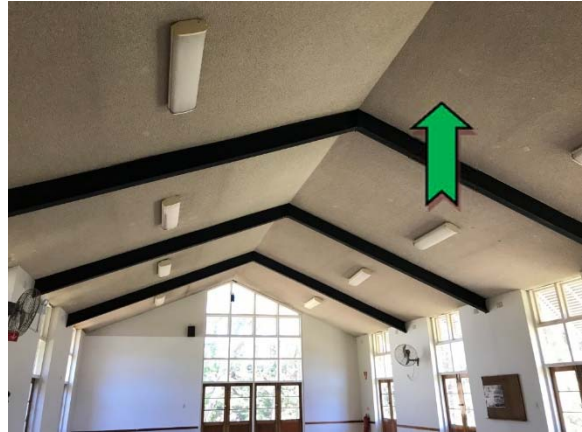
Photo 14. Interior, hall, ceiling, throughout – non asbestos-containing vermiculite.
