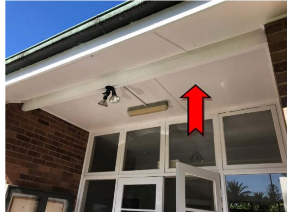
Photo 2. Exterior, eastern elevation, awning – assumed asbestos-containing fibre cement sheeting.
